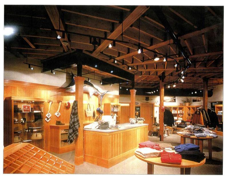
redesigned and exposed. The ceiling was sandblasted and new, heavy floor joist hangers were installed.
